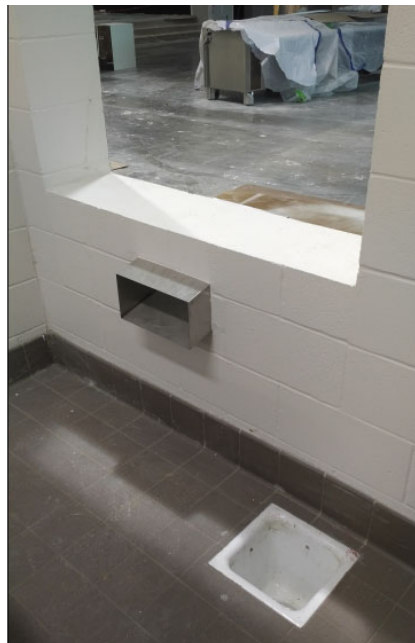
Diagram 11_02 (Refer to Division 11) – Kitchen Chute Tray Detail 2
